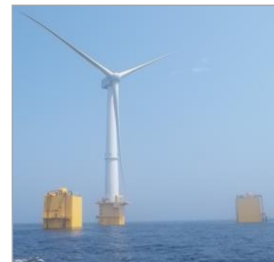
7MW Wind Turbine with DD Transmission
