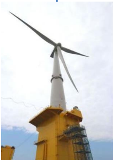
7MW offshore turbine (3.2MW average output)
